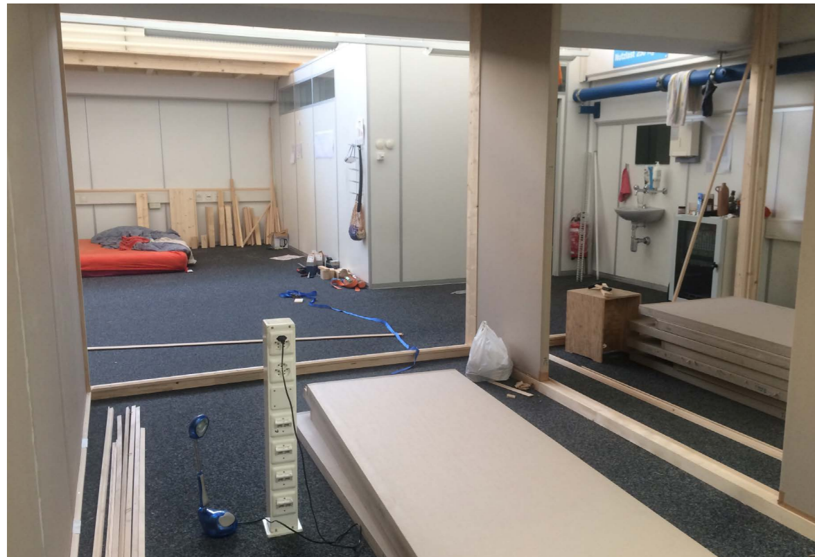
Views of the living and studio space in the former Coop headquarters in Pratteln, Photo: Volume3
